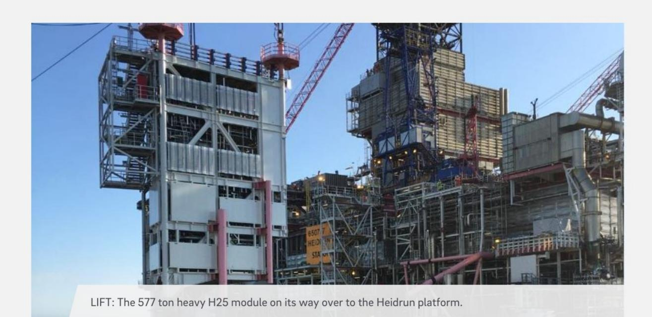
Six days after leaving the yard in Haugesund, the Dvalin H25 module is now installed on the Heidrun platform.
